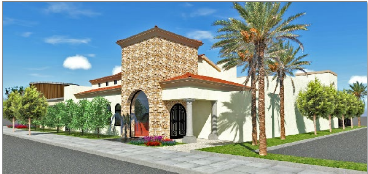
139 West Santa Fe Avenue
