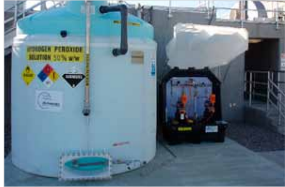
Trojan UV-oxidation solutions include complete H 2 O 2 storage, delivery and monitoring systems that meet the most stringent safety standards.
