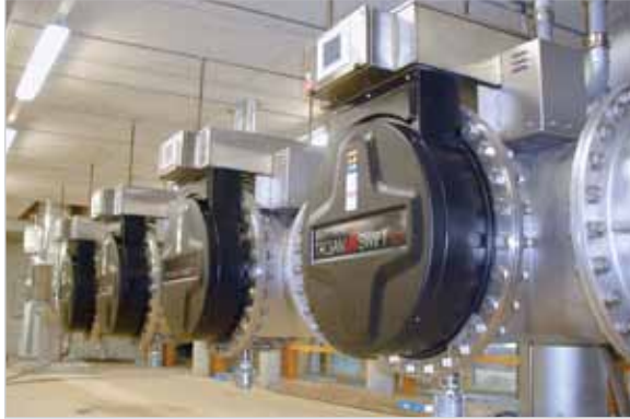
The TrojanUVSwift™ ECT was developed using advanced Computational Fluid Dynamics modeling, resulting in a compact, highly efficient system that minimizes space requirements and installation costs.
