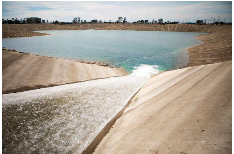
A recharge basin in nearby Anaheim slowly puts water back into the groundwater basin while naturally filtering and purifying it.
