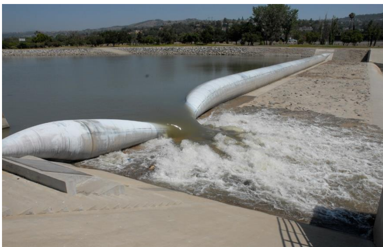
Rubber dams help control Santa Ana River water flows that eventually reach the Orange County Groundwater Basin.
