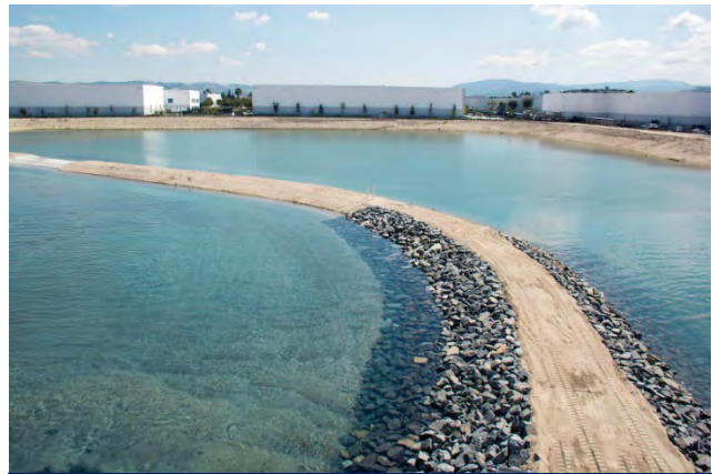
A recharge basin in Anaheim holds water that percolates into the Orange County Groundwater Basin and eventually gets pumped out and distributed to homes and businesses.
