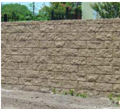
④ Split Face Block Wall with CMU Cap
