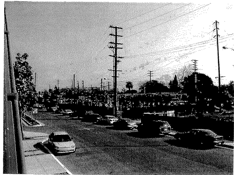
Sub-Station and Walnut Way
