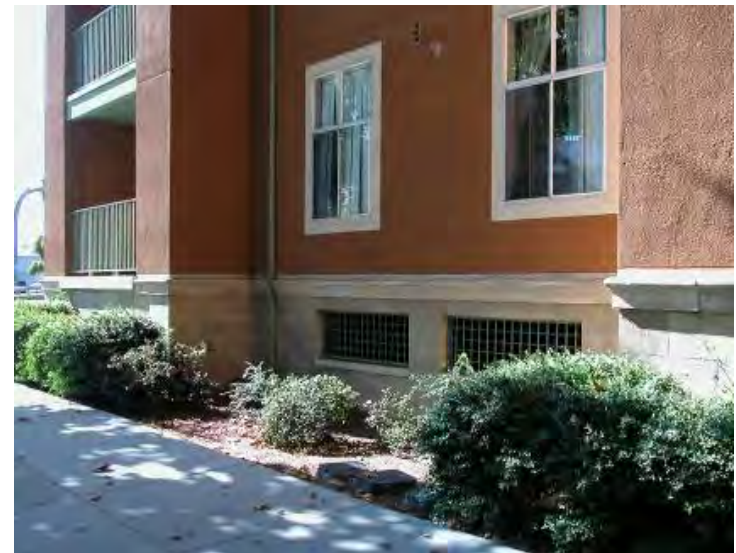
Examples of appropriately designed facades on podium parking levels. The parking levels have facades that are compatible with the rest of the structure and window openings with decorative metal grates to screen views into the structure: allowed
