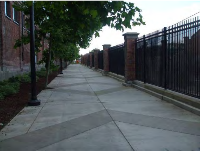
Bike path adjacent to railroad
