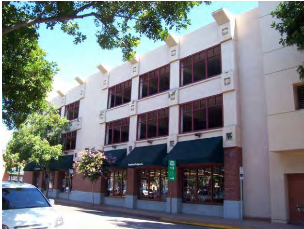
Parking structures that generally comply with standards for parking structure facades: Allowed
