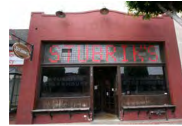
Stubrik's Steakhouse Restaurant Building
