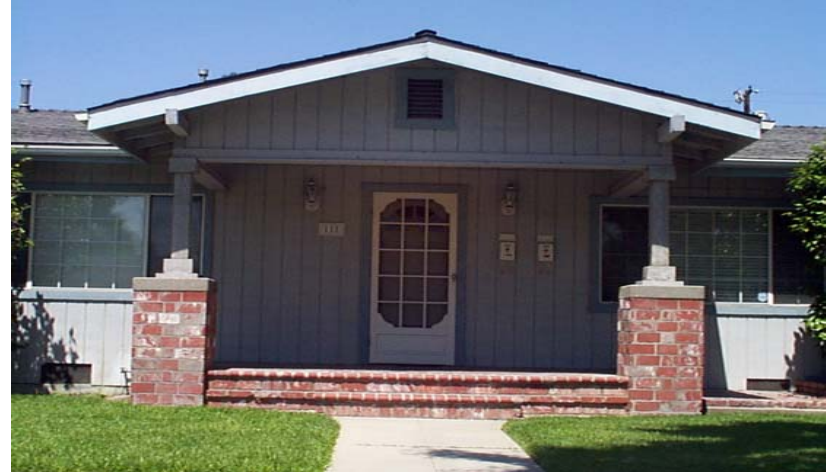
A residence on the 100 block of North Cornell Avenue: a remodel of a 1920s bungalow in 1991, which does not meet the design guidelines. Although well crafted, the new construction includes the use of vertical wood siding, improper design and scale of posts supporting the roof, and the replacement of original windows.
