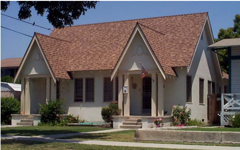
A duplex on the 500 block of North Malden Avenue: it exhibits an appropriate type and color of composition shingle for the mass of the roof.
