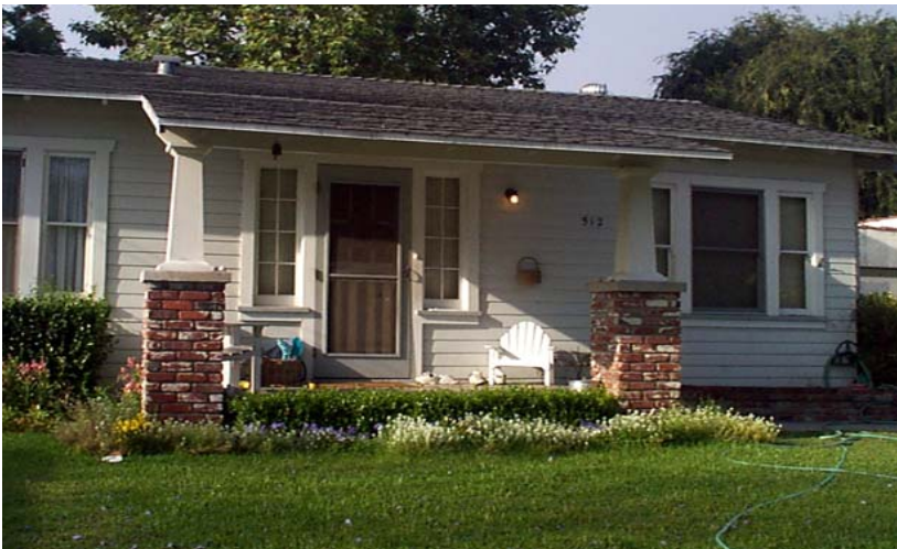
A residence on the 500 block of West Jacaranda Place: the reconstruction of porch supports incorporates appropriate materials, dimension and scale in the design.
