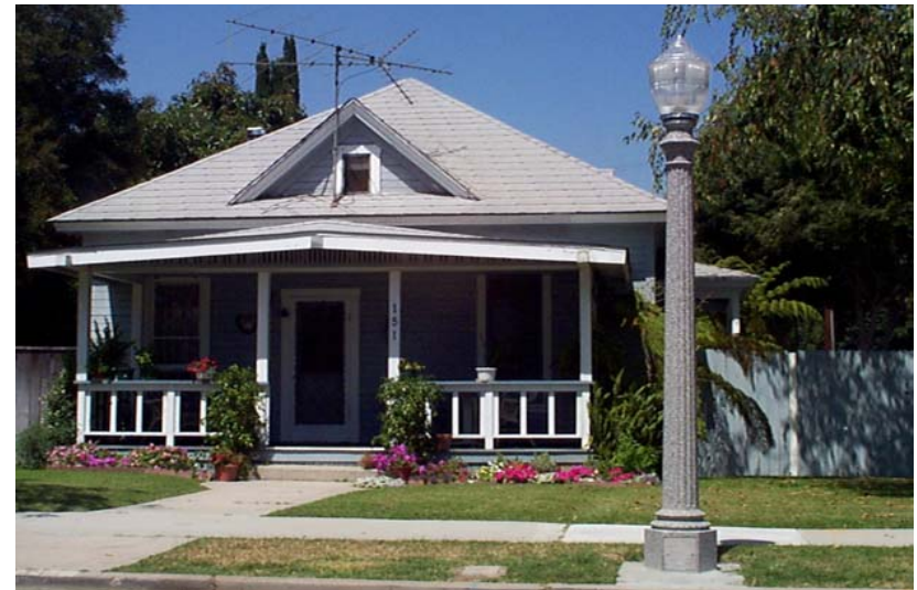
The installation of streetlights on North Lincoln Avenue in 2001: the design and placement of new light standards and lamps respects the historic nature of this neighborhood.
