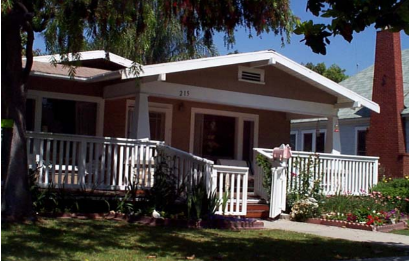
A residence on the 200 block of North Berkeley Avenue: a good design of a railing to enclose a porch of a Craftsman bungalow.
