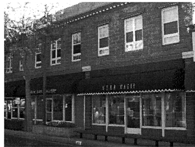
The quality of workmanship for the exterior treatment is as important as the design.
